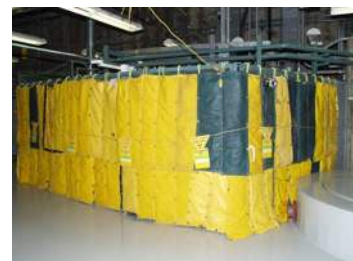
Lead Blankets as Shielding
